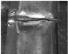
Rupture de rail
